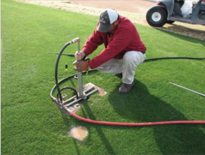
Figure 2. The simple act of raising and leveling sprinklers can improve system efficiency by as much
